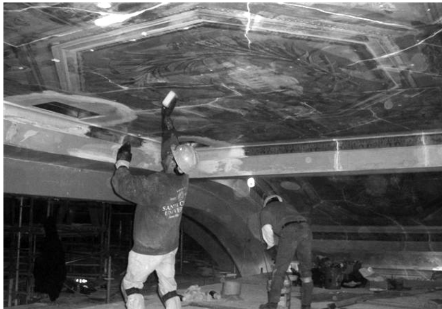
EVERGREENE STUDIOS WORKING ON CEILING
