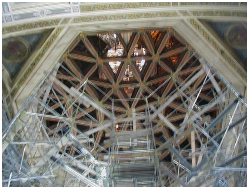
DOME UNDER CONSTRUCTION
