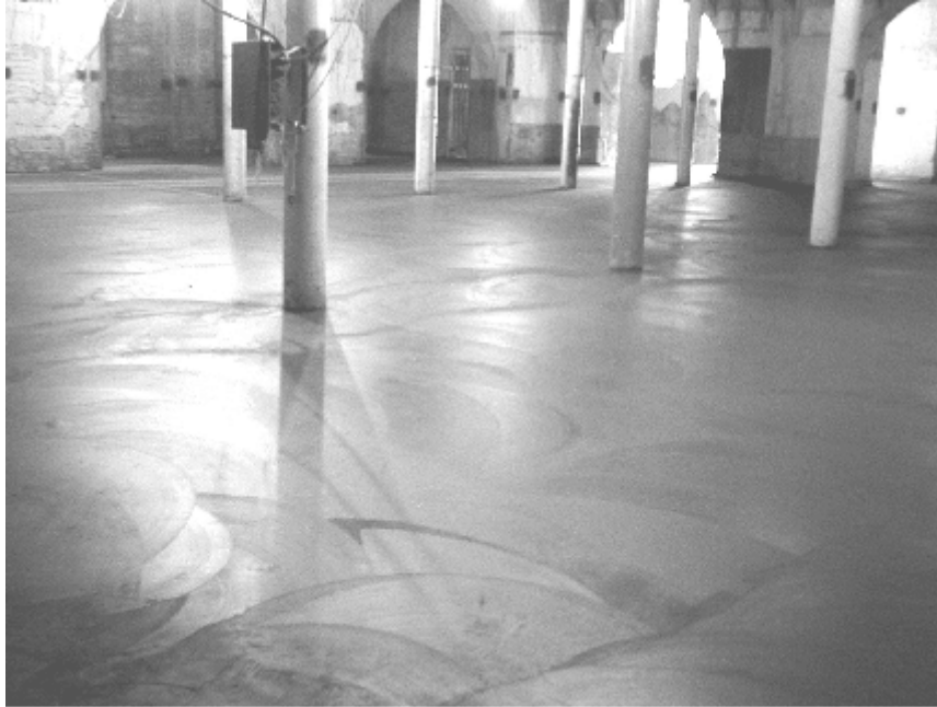
NEW LOWER LEVEL CONCRETE FLOOR
